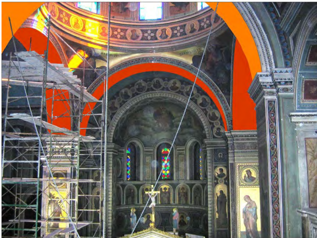
Figure-16: Placement of CFRP on the arcs of central dome
