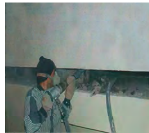
Figure 11: The views of a two-stage system of R/C continuous beams, which separate the building from its foundation and create the seismic isolation system
