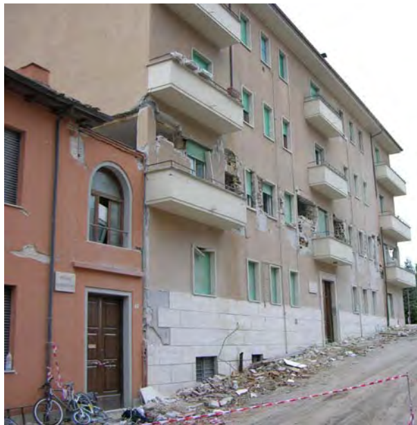
Figure 1: Damage of a four-story conventional building due to pounding with its adjacent two-story building, during the L'Aquila earthquake in Italy, in April 2009
