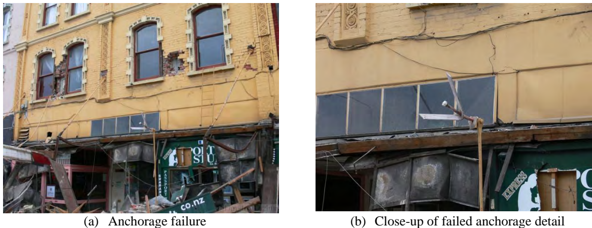
Figure 3: Anchorage failure of awning brace due to parapet collapse.
