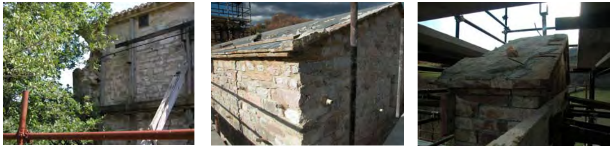
Figure 25: The Santa Croce della Ficarella Church in Case Basse (Perugia) put in safe conditions after the 1997-98 Marche & Umbria earthquake (left) and subsequent conventional restoration works (at the centre and right), which should have been followed by the construction of a sub-foundation and insertion there of a SI system formed by 8 HDRBs with 600 mm diameters and 294 mm height (maximum design displacement = 256 mm).
