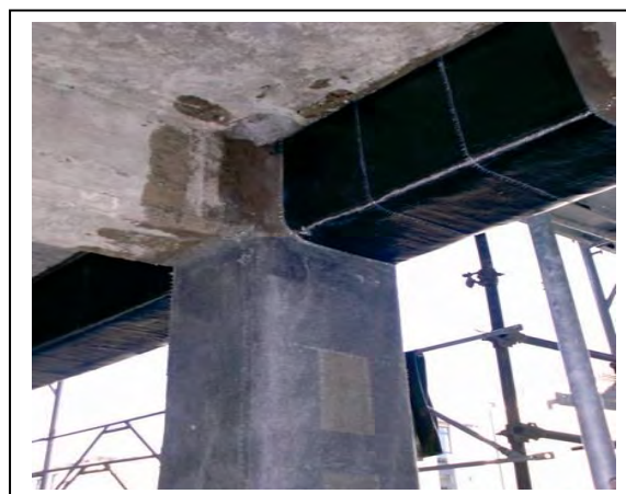
Fig.23- Example of old concrete rehabilitation using thermo welded Betontex unidirectional carbon reinforces.
