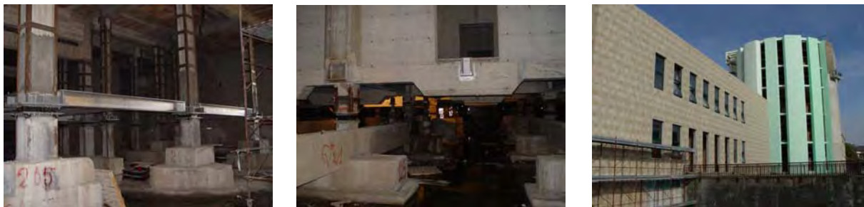
Figure 8: Installation of the steel beams floor in the building of Figure 6 just above the isolators and reinforcement of the pillars (left); the lower floor after cut of the building supporting pillars and walls (at the centre); the building after retrofit completion (right).
