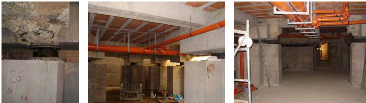
Figure 19: A HDBR installed, after demolition of the parts of the original foundation piles which were not encompassed by the new pillars (left); the new underground floor in the aforesaid conditions and after the installation of the pipe lines (at the centre and right).
