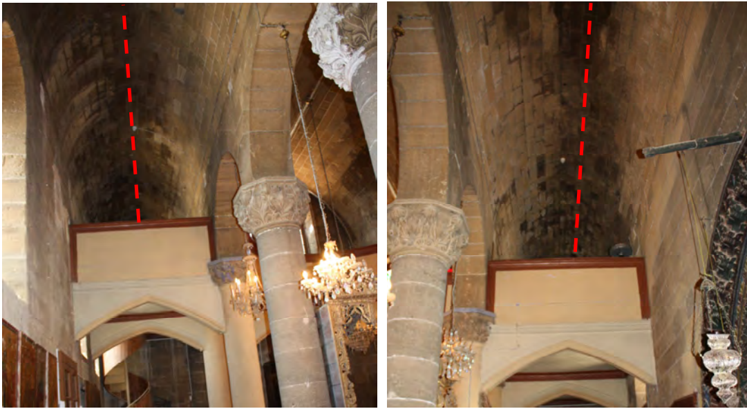
Figure 2: Pictures depicting two aisle vaults along which the lowest temperatures within the structure were detected.
