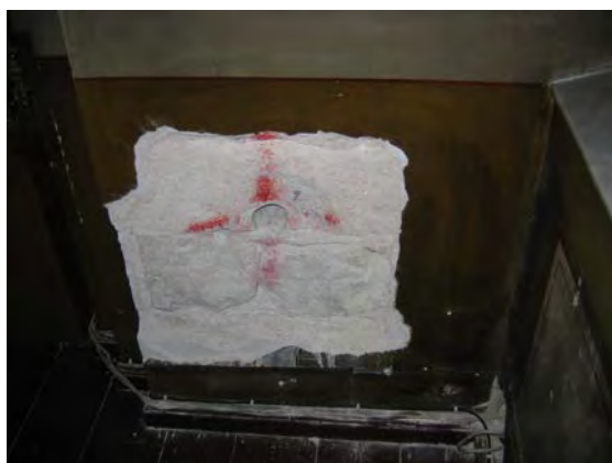
Figure-5: Area without mortar cover
