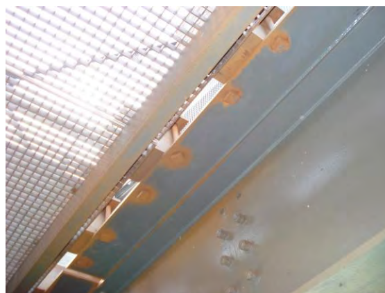
Figure 13: Sleepers-longitudinal girder connection by catch bolts
