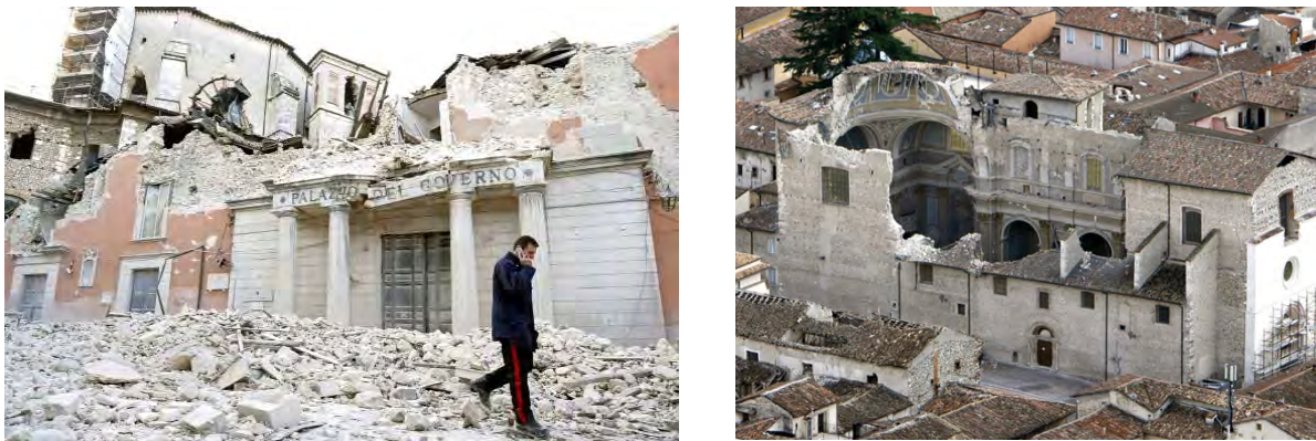
Figure 3: The Prefettura building (provincial headquarters of the national government) of L'Aquila, a symbol of lack of prevention of the seismic risk in Italy until 2009 (left), and the Santa Maria Paganica Church (right), collapsed after the 2009 Abruzzo earthquake.
