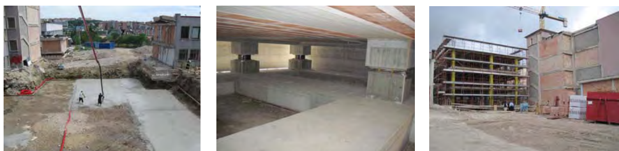
Figure 39: The Romita High School in July 2010, after the demolition of blocks "A" and "B" (left); two HDRBs and a SD installed in the underground technical floor of the new block "B" of the school, during its reconstruction (at the centre); state of the reconstruction of the new block "B" in October 2010, before casting of the upper deck, at the side of the original block "C" (right).
