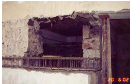
Figure 9: The views of the lower reinforcement frames of the lower pedestal installed in the opening together with the isolator socket
