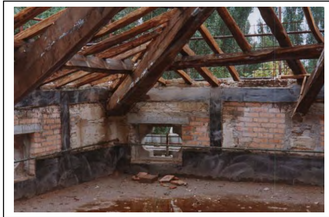
Fig.24- Example of building complete belting ( inside and outside ) , at Villa Bertani- Reggio Emilia damaged by earth quake of 1996 , using thermo welded Betontex unidirectional carbon reinforces.
