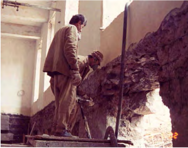
Figure 8: Retrofitting of existing 3-story stone school building: the case when the opening has the part of the existing wall above it
