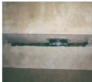
Figure 11: The views of a two-stage system of R/C continuous beams, which separate the building from its foundation and create the seismic isolation system
