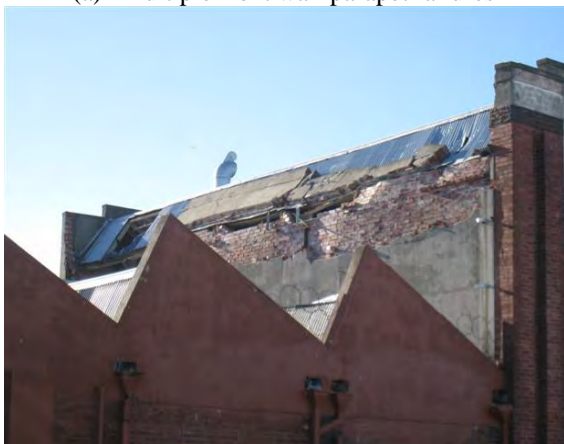
(c) Side wall parapet collapse onto roof.
