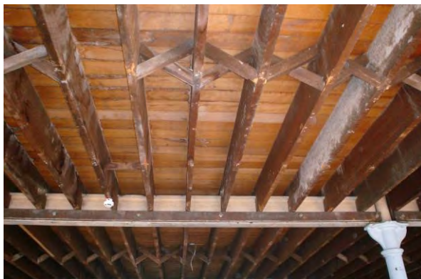
(a) Underside showing joists, sheathing and cross-bracing
