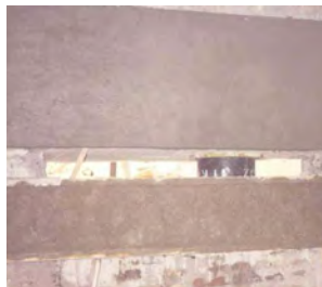
Figure 11: The views of a two-stage system of R/C continuous beams, which separate the building from its foundation and create the seismic isolation system
