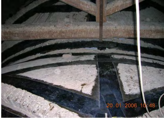
Fig.21- Example of extrados vaults reinforcement by carbon fibres tapes, (S. Giorgio Church, near Bologna-Italy)
