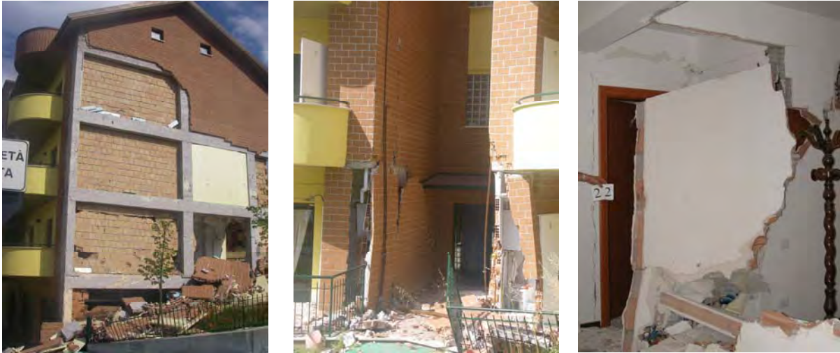
Figure 35: Damage caused by the 2009 Abruzzo earthquake to the building of Figure 34; its retrofit by means of HDRBs and SDs has been planned, based on a design of the already mentioned GLIS and ASSISi member G. Mancinelli of Fabriano, with safety certification of A. Martelli.
