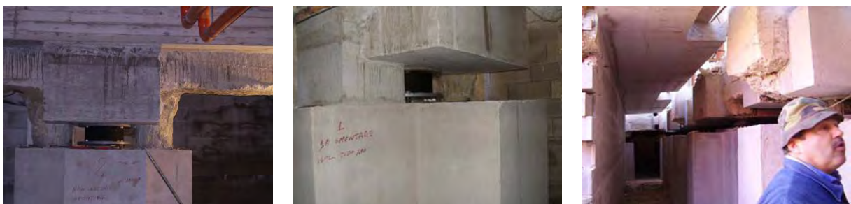
Figure 18: HDRBs installed between two original (left) and two newly built (at the centre) foundation piles of the house of Figure 11, before demolition of their parts which were not encompassed by the new pillars; the underground floor after demolition of the aforesaid parts (right).
