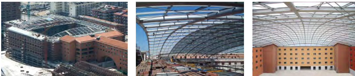
Figure 22: New ceiling of the Crowne Plaza Hotel in Caserta, set up by the GLIS board member and ASSISI member G.C. Giuliani of Milan in 2006 by constraining it by means of SDs to 3 of the 4 buildings to which it is connected.
