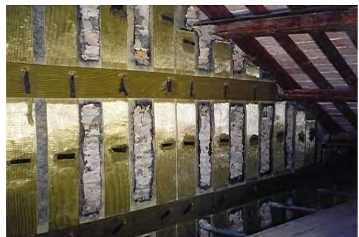
Fig. 20 -Inside walls reinforcement of Tympanum of Library.
