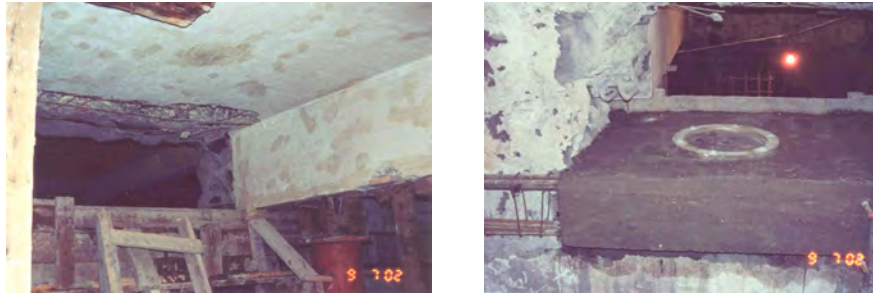
Figure 12: Existing beam is crossing the space of the opening and supported by temporary columns
