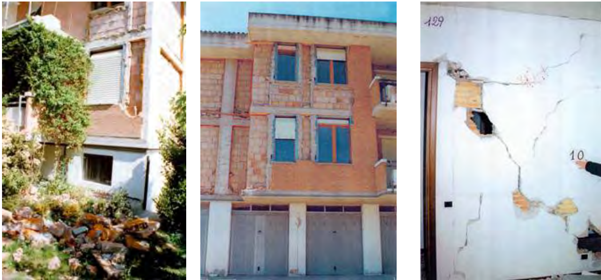
Figure 12: External and internal non structural damage suffered by the house of Figure 11 in the 1997-98 Marche & Umbria earthquake.
