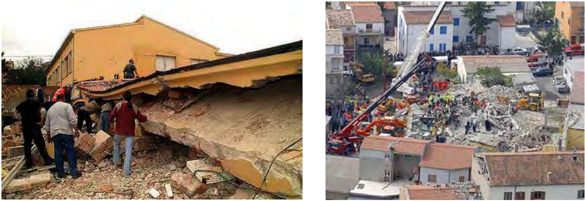
Figure 2: Collapse of the Francesco Jovine primary school of San Giuliano di Puglia (Campobasso) during the 2002 Molise & Puglia earthquake and search of survivors amid the debris. Prior to the aforesaid earthquake the San Giuliano di Puglia area was not seismically classified (now it is classified in seismic zone 2).
