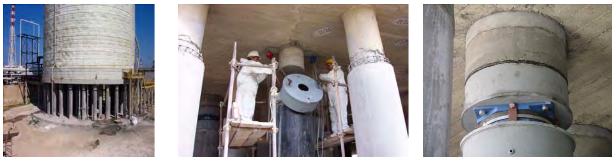
Figure 23: One of the 3 tanks of Polimeri Europa located in Priolo Gargallo (Augusta, Syracuse, seismic zone 2*), which were seismically retrofitted using U.S. FPS devices in the years 2005-2008 and one of the isolators during and after its installation.
