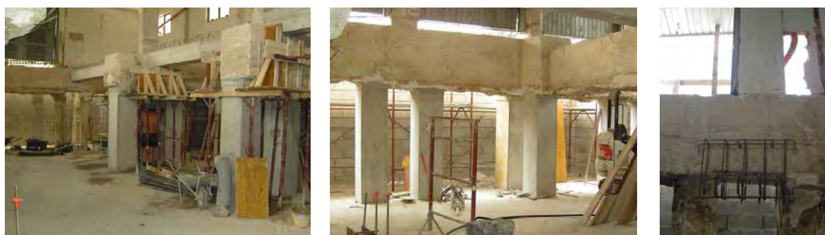
Figure 14: Newly built foundation piles, in the part of the house of Figure 11 where the original ones were failing (left and at the centre); pillar eccentric with respect to the original foundation piles (right).
