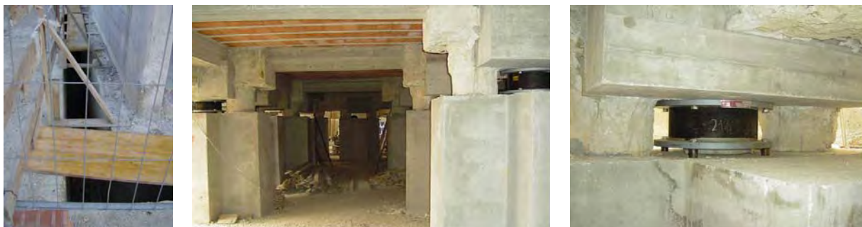
Figure 17: Lateral structural gap of the house of Figure 11 before the installation of its protection plates (left); the new underground floor after installation of the HDRBs, but before demolition of the parts of the original foundation piles which were not encompassed by the new pillars (at the centre); an installed HDRB superposed to an epoxy flat jack (right).
