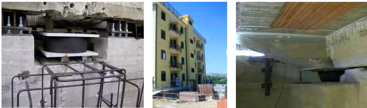
Figure 10: A HDRB during its installation in one of the buildings of Figure 9 (left); this building after retrofit completion (at the centre); an isolator laterally deformed during the on-site tests (right).
