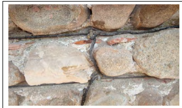
Fig.10. Historical City Walls in stones ( Bassano- Italy), reinforced with hybrid aramid – carbon fibres cable, prestressed and impregnated with epoxy resins. Courses among stones will be filled by traditional mortar.
