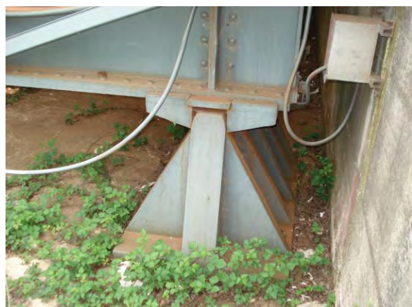
Figure 11: General view of fixed bearing
