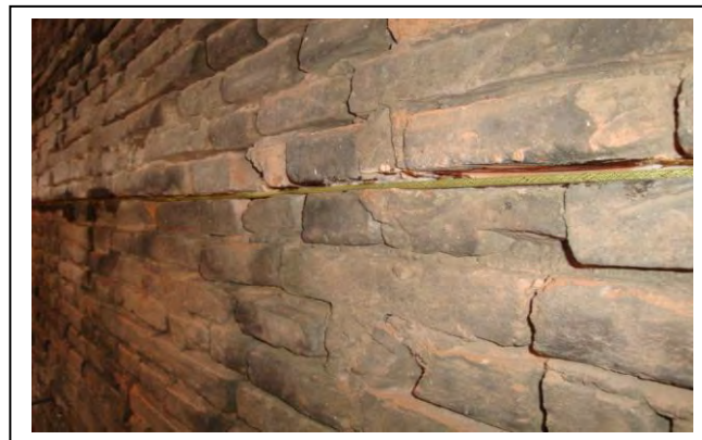
Fig.11. Bricks walls reinforced with carbon fibres cable coated with aramid fibres, prestressed and impregnated with epoxy resins. Courses among bricks will be closed by traditional plaster.
