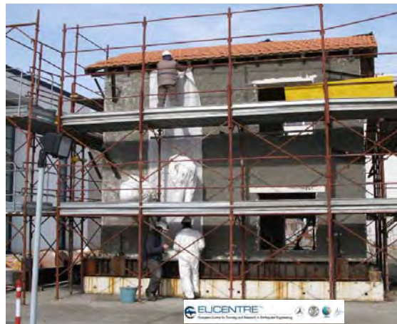
Figure 9: Masonry building with textile application
