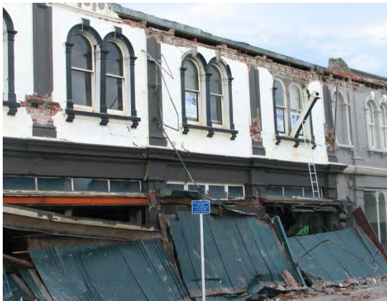
(a) Multiple front wall parapet failures
