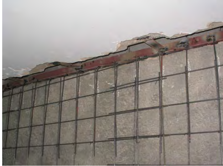
Figure 10. A typical view of the intersection between enhanced bearing walls and floor slab.
