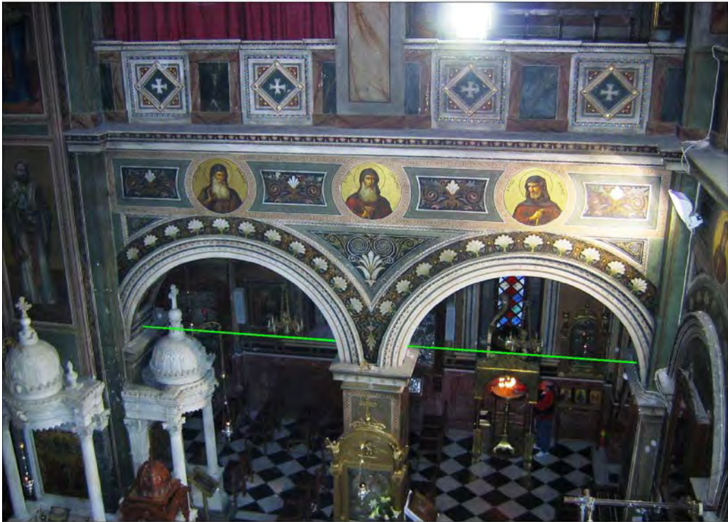
Figure-17: Placement of tie rods at arcs
