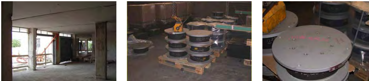
Figure 16: New r.c. slab of the ground level floor of the house of Figure 11 (left); the HDRBs before their installation in the new underground floor (at the centre and right).
