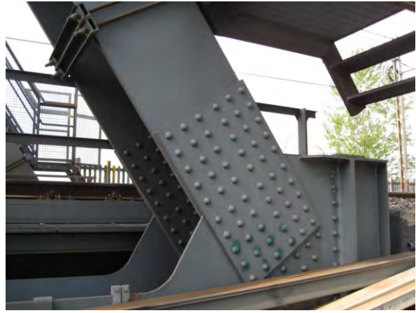
Figure 7: Riveted diagonal-lower string joint of Panaro bridge
