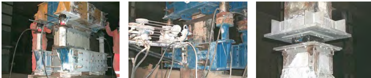
Figure 7: Phases of the retrofit of the building of Figure 6, with installation of 4 hydraulic jacks to provisionally support the weight after removal of the pillar part to be replaced by an isolator and to locally lift the building, so as to allow for the subsequent insertion of the isolator (left), and cut of the pillar with a linear saw (at the centre); view of the isolator after its installation and its mechanical fixing to the upper and lower pillar parts (right).
