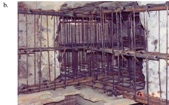
Figure 10: The view of the isolator installed in the socket after casting the concrete of the lower pedestal (a), and of the upper reinforcement frame installed in the opening together with the upper socket and with the binding reinforcement upper frames (b)
