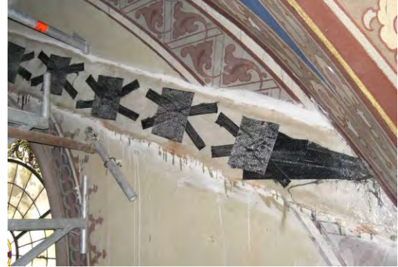
Fig.22- Example of walls reinforcement using Ard-fix connectors, at Alba Cathedral in Cuneo- Italy.
