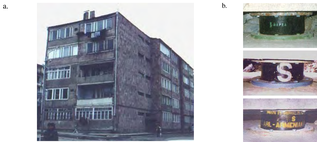
Figure 1: General view of the retrofitted by base isolation existing 5-story stone apartment building (a) and a fragments of its isolation system (b)
