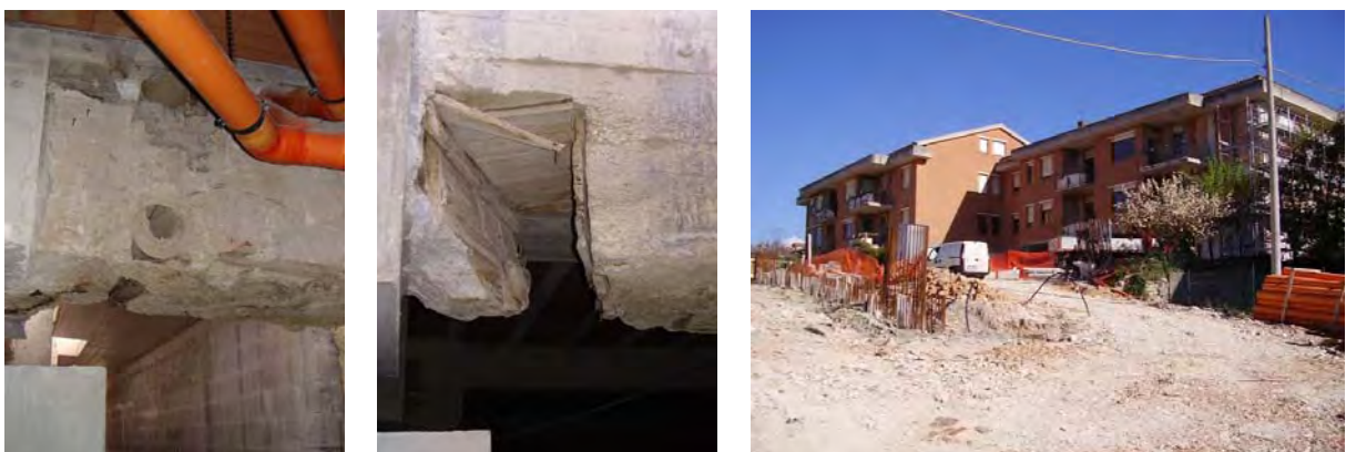
Figure 20: Holes and breaks in the beams of the house of Figure 11, made during the initial construction to create passages for the pipe lines (left and at the centre); the house after retrofit completion (right).
