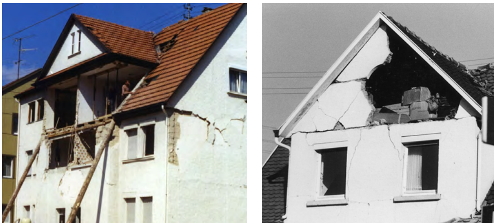
Figure 1: Out-of-plane failure after the earthquake in Albstadt, Germany, 1978 (Photos: Peter Doll)
