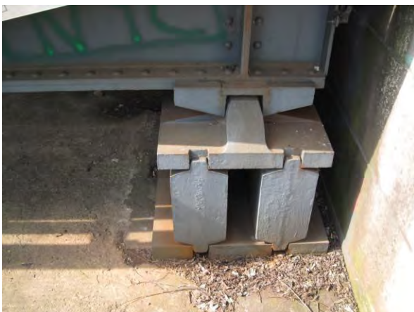
Figure 10: General view of unidirectional bearing
