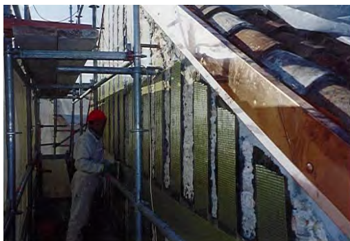
Fig. 19 -Outside walls reinforcement of Tympanum of Library .
