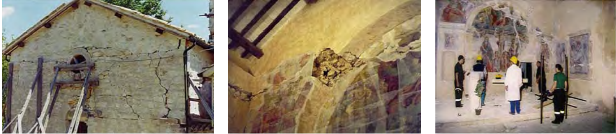
Figure 24: External and internal damages suffered by the San Giovanni Battista Church in Apagni (Perugia) during the 1997-98 Marche & Umbria earthquake.
