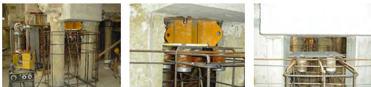
Figure 15: Setting up of the reinforcement of the lower stump of the new pillar (by means of a dummy isolator) and of the lower plate for connecting the isolator in the new underground floor of the house of Figure 11.
