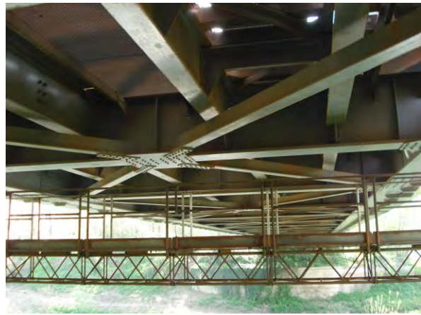
Figure 9: General view of lower and track bracings
