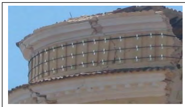
Fig.9. Application of Betontex Aramid Tie 85 HM on the tambour of “Anime Sante” Cathedral, L’Aquila, damaged by earthquake of 2009. The Tambour was put in security to proceed with further works.
