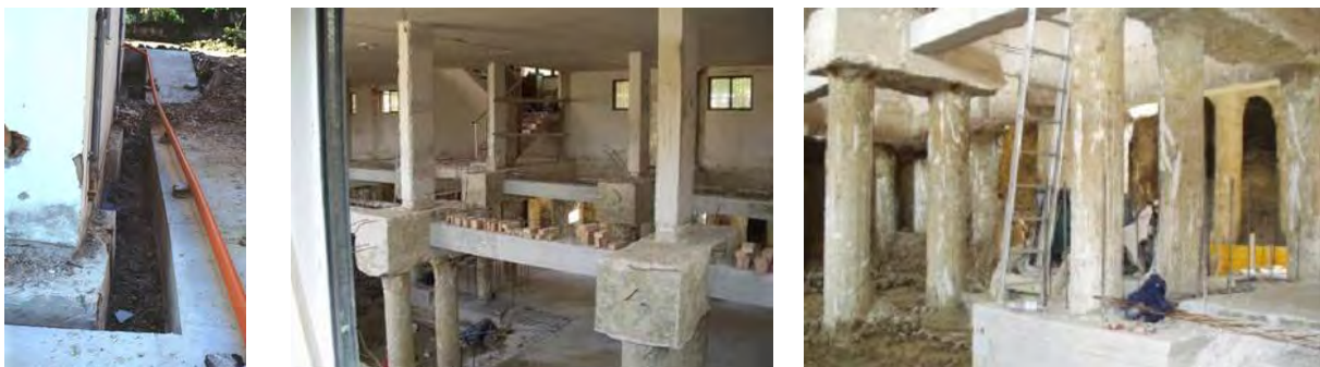
Figure 13: Creation of the structural gap around the house of Figure 11 (left); view from the top of the original lower floor and the new underground one after excavation of the latter and construction of new curbs (at the centre); view from the bottom of the new underground floor, the original foundation piles and the new foundations under constructions (right).
