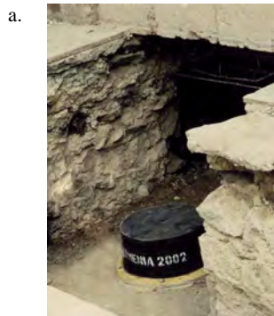
Figure 10: The view of the isolator installed in the socket after casting the concrete of the lower pedestal (a), and of the upper reinforcement frame installed in the opening together with the upper socket and with the binding reinforcement upper frames (b)
